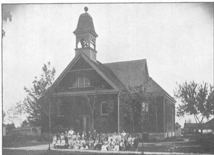
EAST PRIMARY BUILDING.
